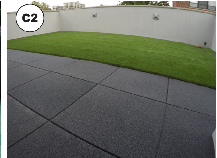
C2 Turf-top Rubber Tile for library, meditation, and gaming area Manufacturer: Unity Surfacing Systems Turf-top: 1167 SF
